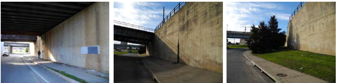
This series of photos depicts the walking experience between the site and downtown. The route is difficult, unappealing, and unsafe for pedestrians and those using other forms of active transportation.
